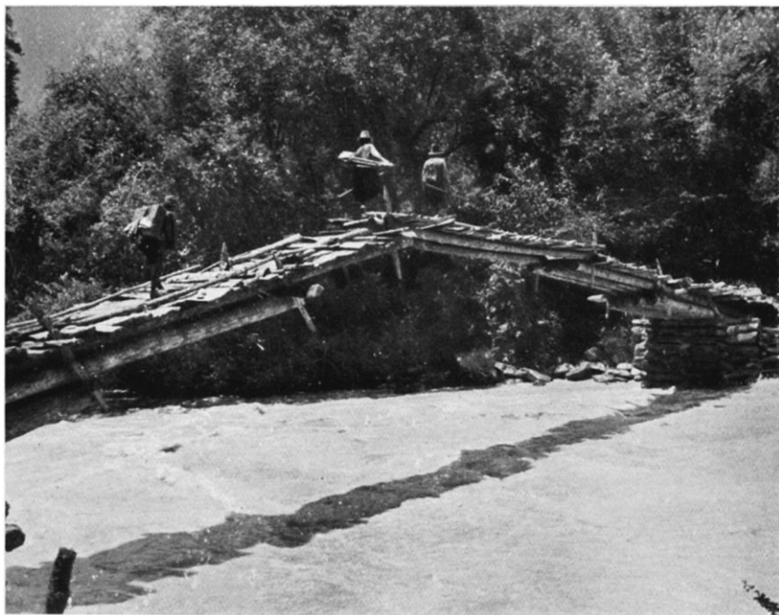
Cantilever bridge near Modung
